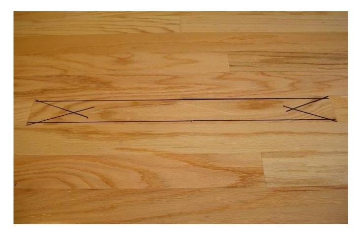
With a marking pen, mark the areas to be cut approximately ½" from the side joints
