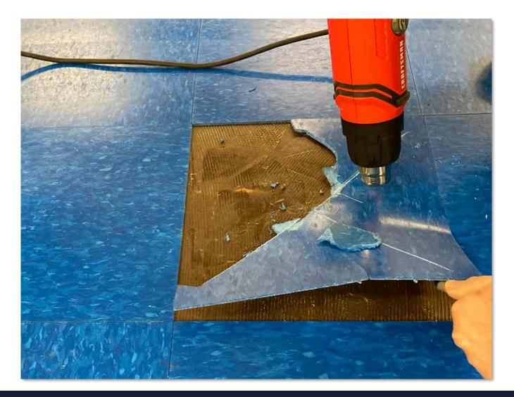
• Continue using heat gun and scraper and work toward the edge as tile softens.
