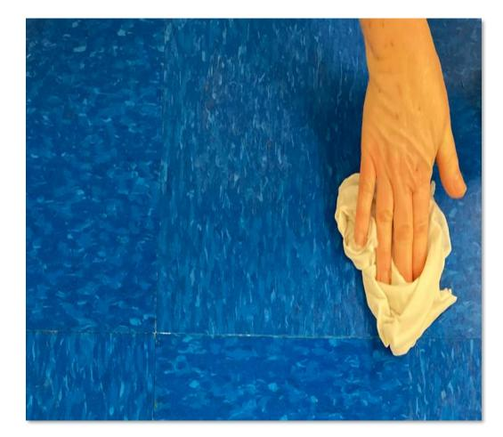
• Clean up adhesive residue and hand roll the tile to ensure proper contact between the adhesive and tile.
