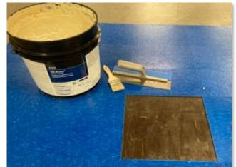
• Spread the VCT adhesive with a fine-notched trowel or a paint brush.
