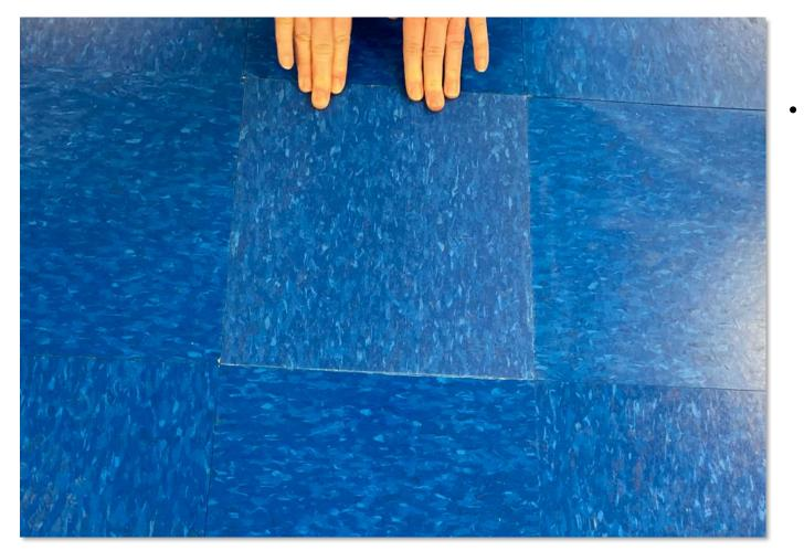
Position tile into adhesive, adjusting as needed.
