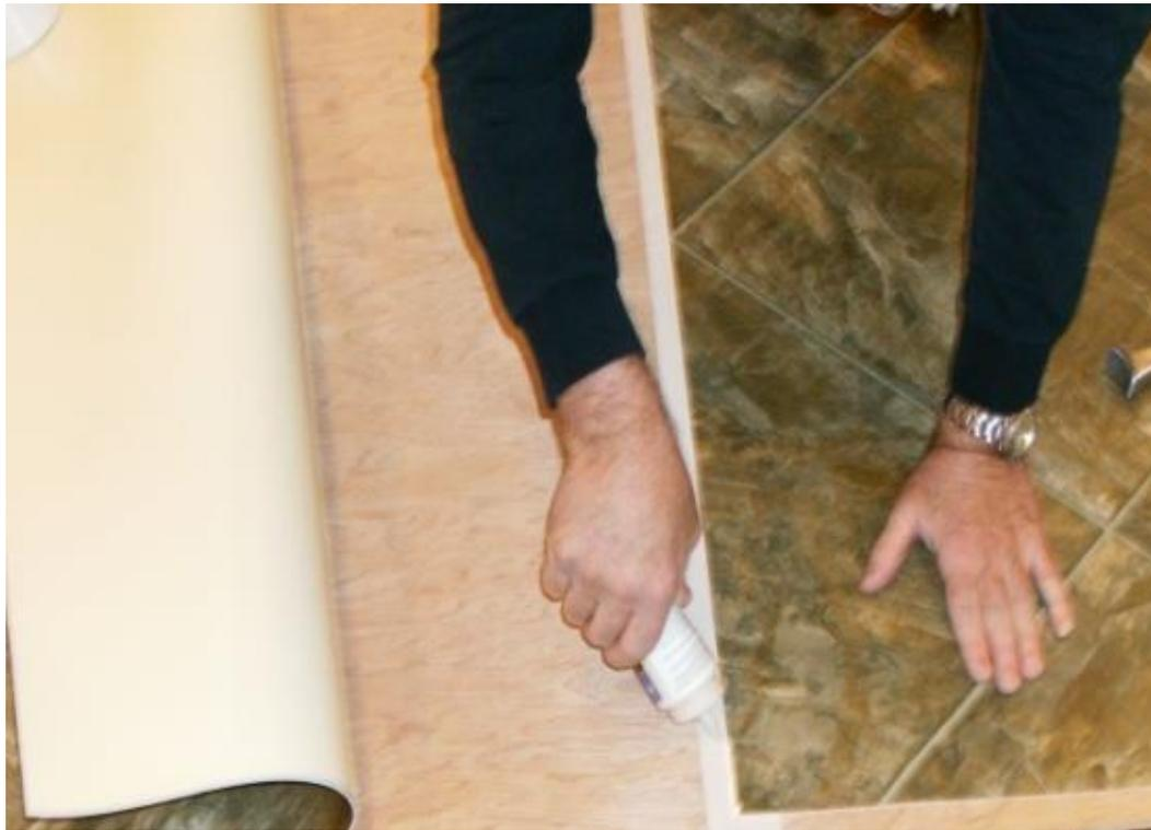
Lay in second piece and hand roll. Adhesive will ooze up between the pieces.
